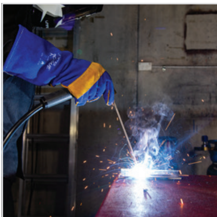
(6) Hold the electrode slightly above the work maintaining the arc while travelling at an even speed.
